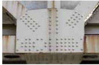
Figure 1: Gusset plate at joint.
