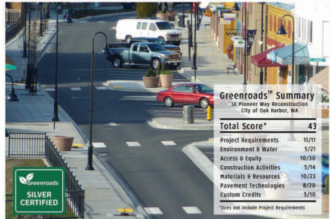
Greenroads Silver Certified project in Oak Harbor, WA. Photo courtesy of Greenroads™ Foundation.
