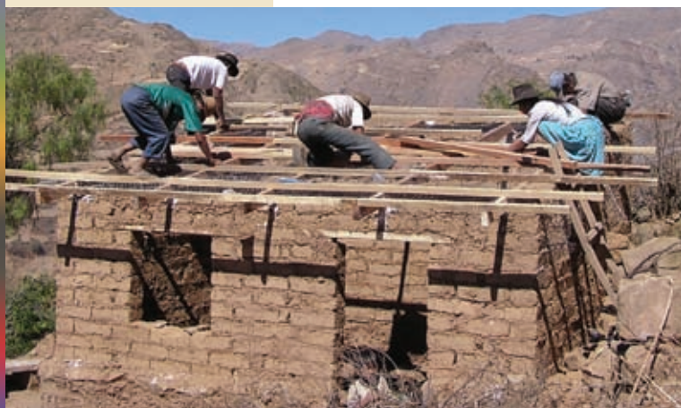
In the village of Yanayo Chico, a team of locals installs the framework for a corrugated metal roof. EWB designed the roof and provided the materials.
