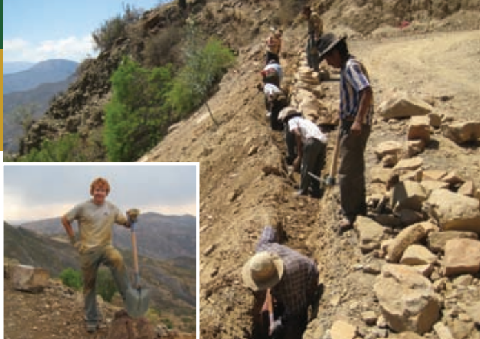
Mountain road repair is a strenuous, dirty job. CEE graduate student Mark Raleigh (inset) helped guide the work done by the village men.
