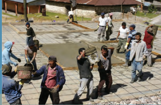
Top left: Children excitedly try out new concrete bleachers, which will hold several hundred people during town meetings and events.
