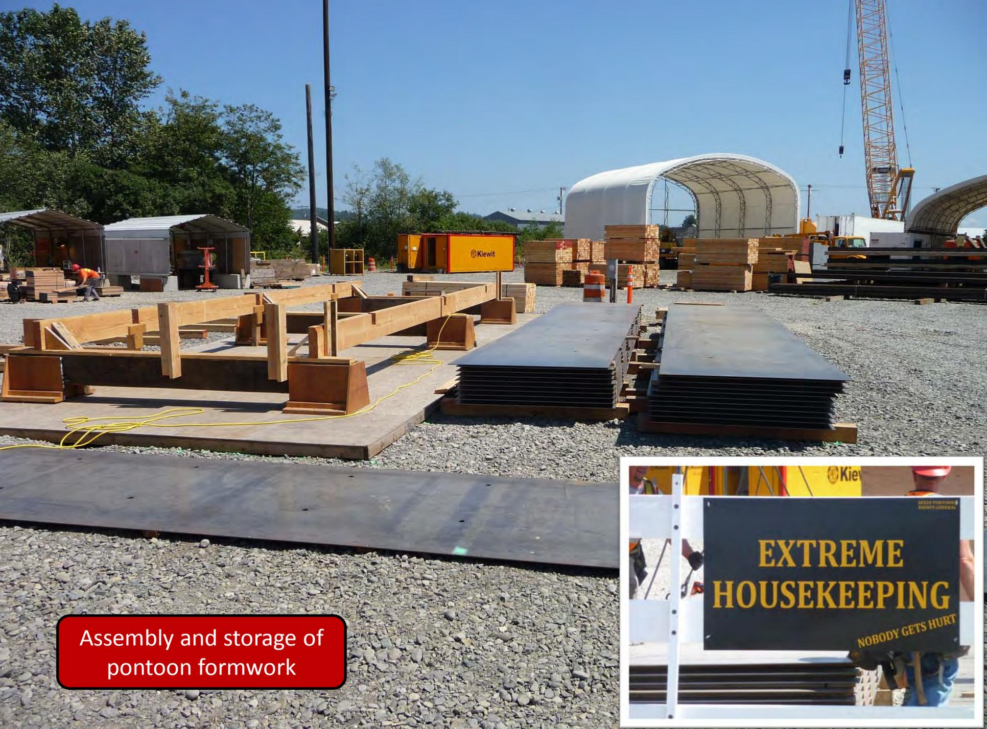
Assembly and storage of pontoon formwork
