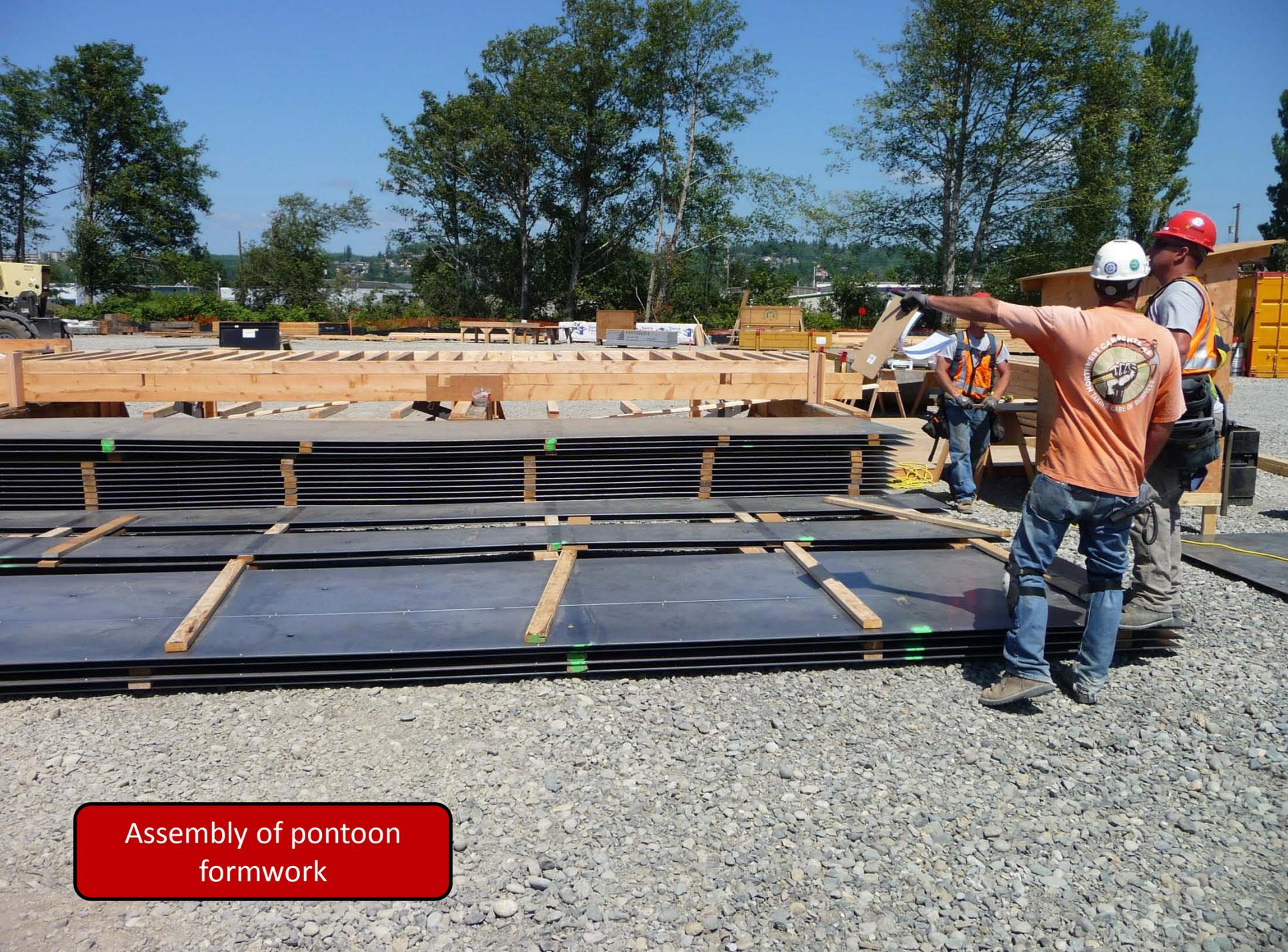
Assembly of pontoon formwork
