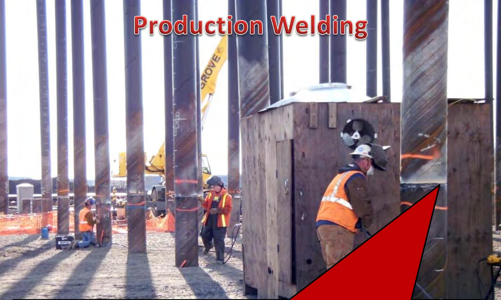
Initial 18" diameter piles to support the casting basin slab had a 70 ft. length. These were driven with about 5 ft. remaining (as shown here). Then an additional length of 65 ft. were welded on (total length 135 ft.) and driving continued. Purpose was to drive from the existing surface prior to major excavation given the poor underlying soil conditions.
