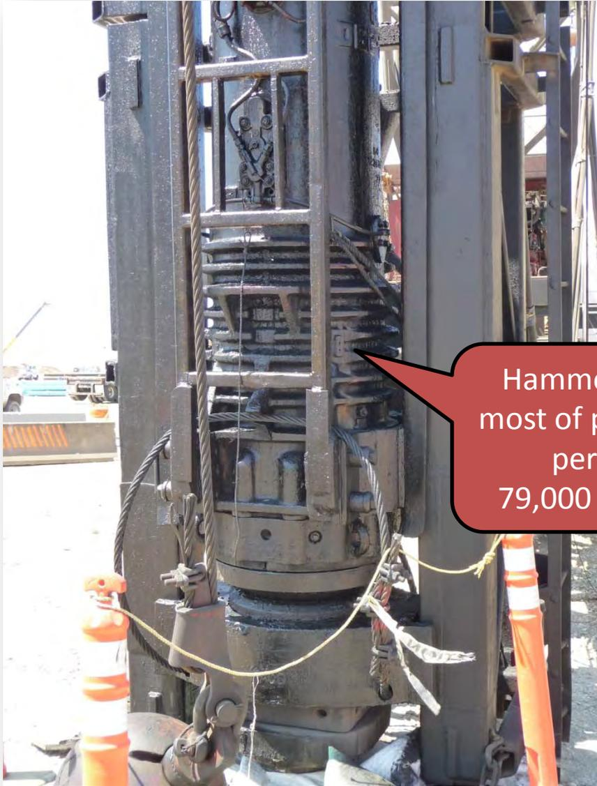
Hammer used to drive most of pipe piles. Energy per blow range 79,000 to 165,000 ft-lb
