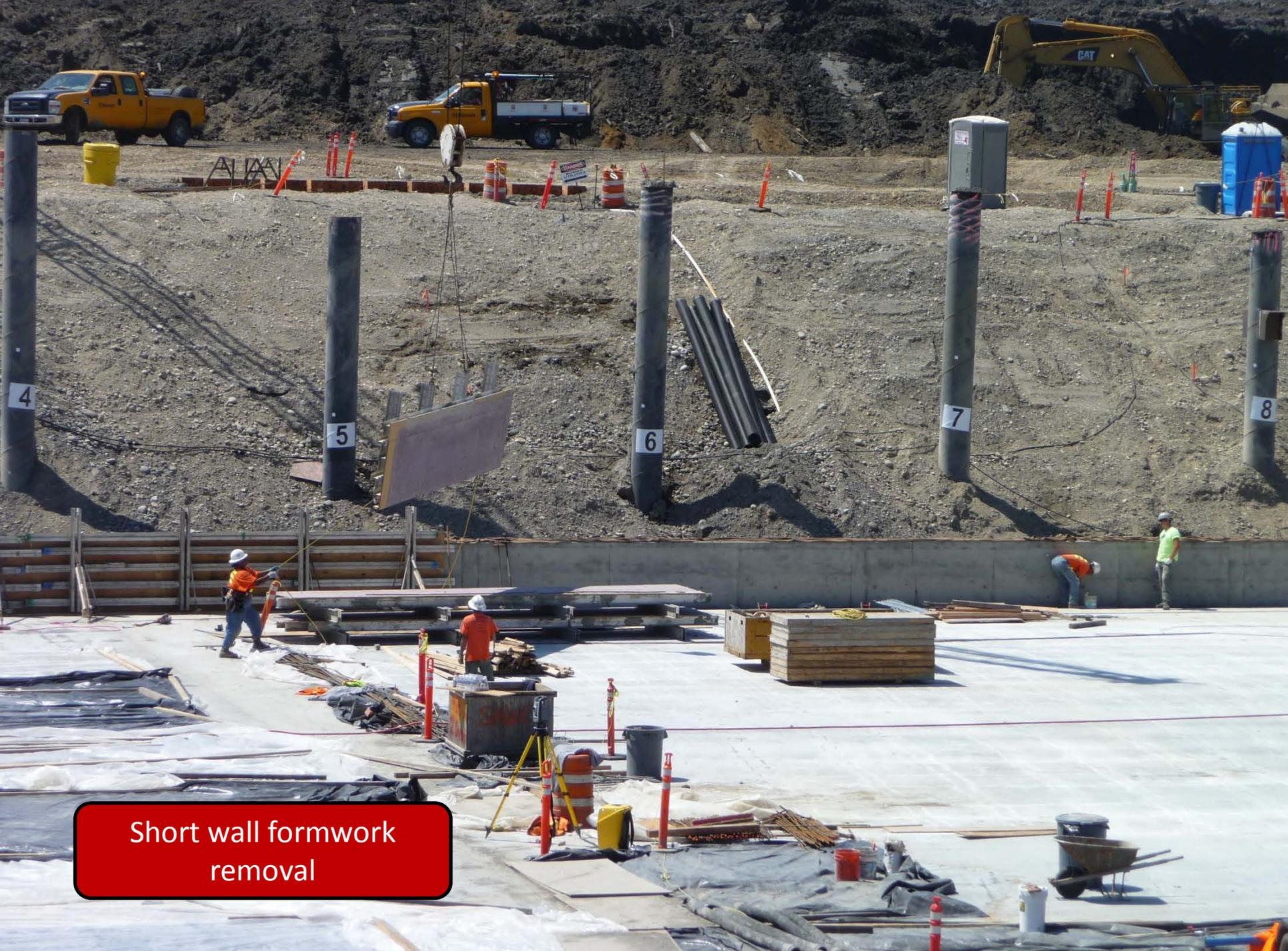
Short wall formwork removal
