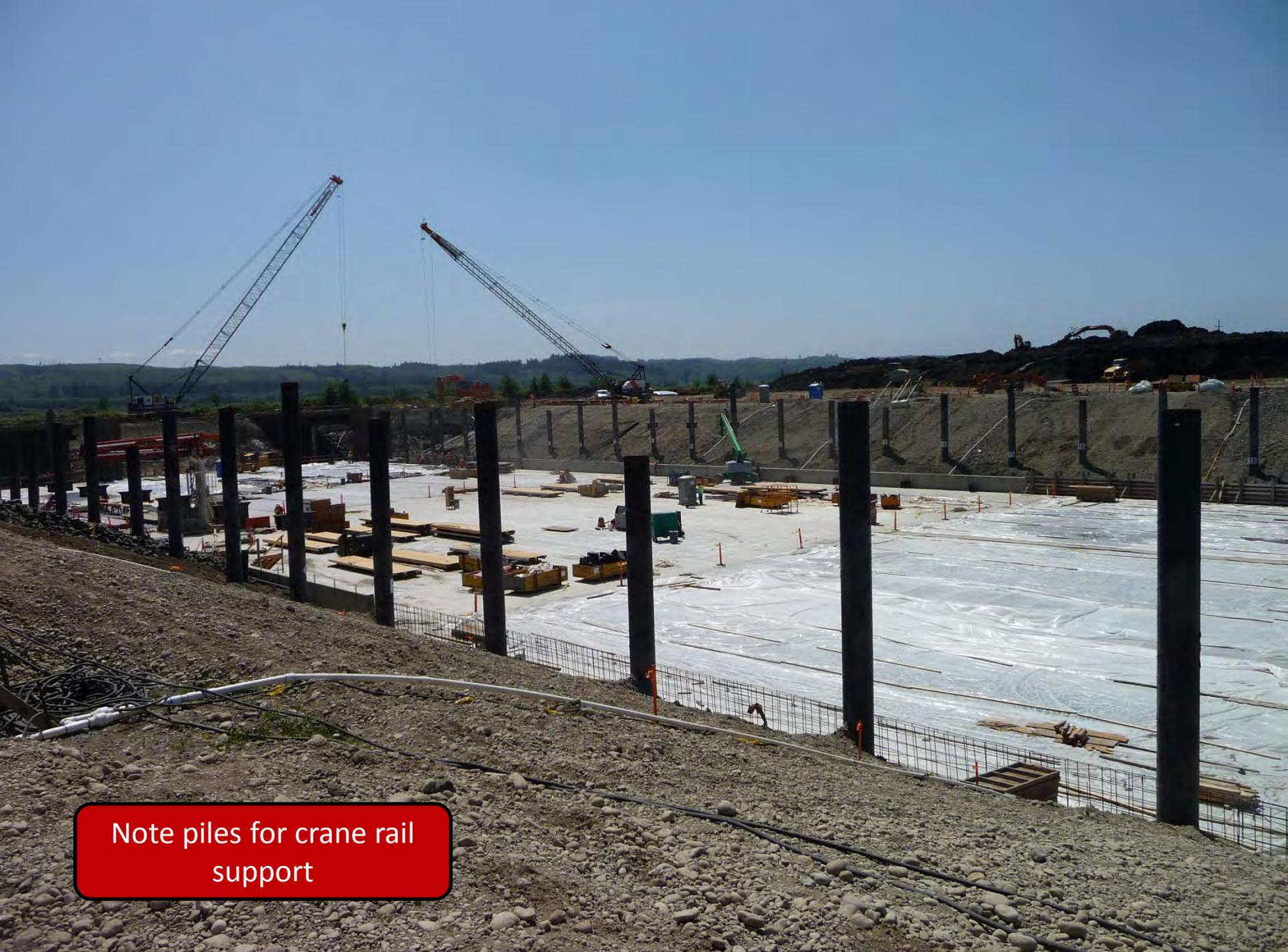
Note piles for crane rail support
