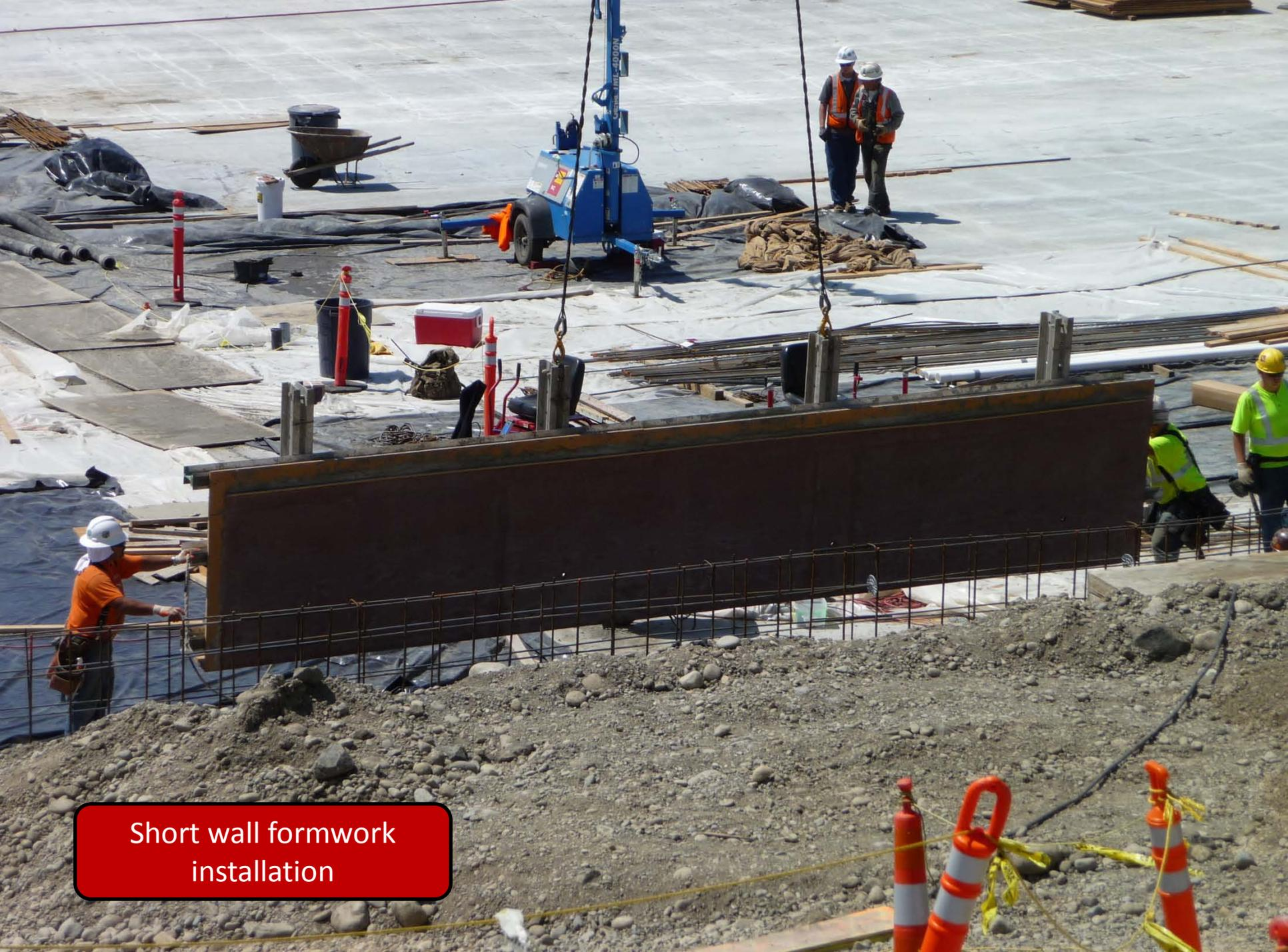
Short wall formwork installation
