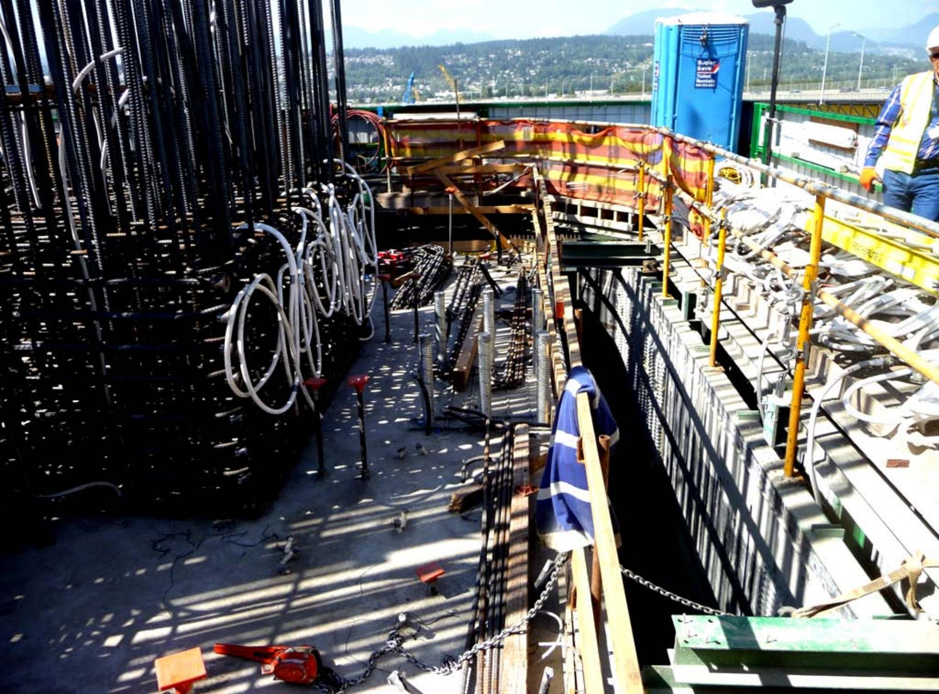
Cooling tubes which use river water. Concrete placed in pylon is defined as mass concrete and must be cooled during early curing. Following sufficient cure time, tubes are grouted closed.
