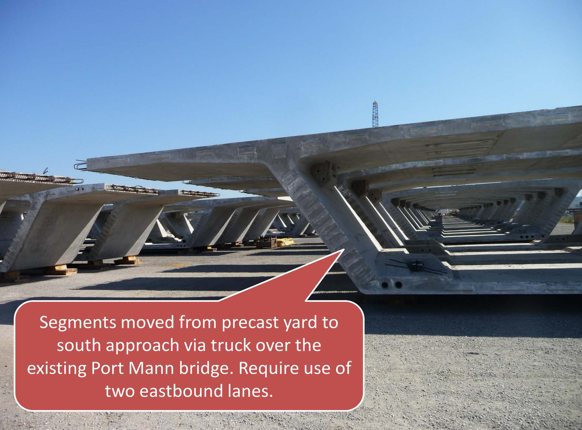
Segments moved from precast yard to south approach via truck over the existing Port Mann bridge. Require use of two eastbound lanes.
