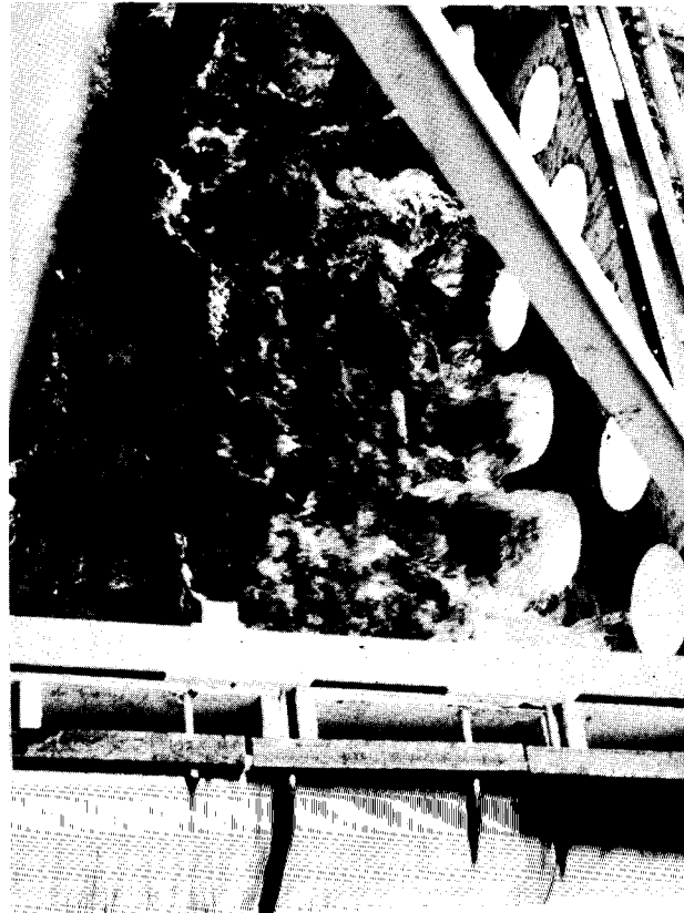
Figures 6 & 7 Breakwater Operation. (Incident wave energy converted to kinetic energy [jets] and dissipated through turbulent mixing and diffusion.)
