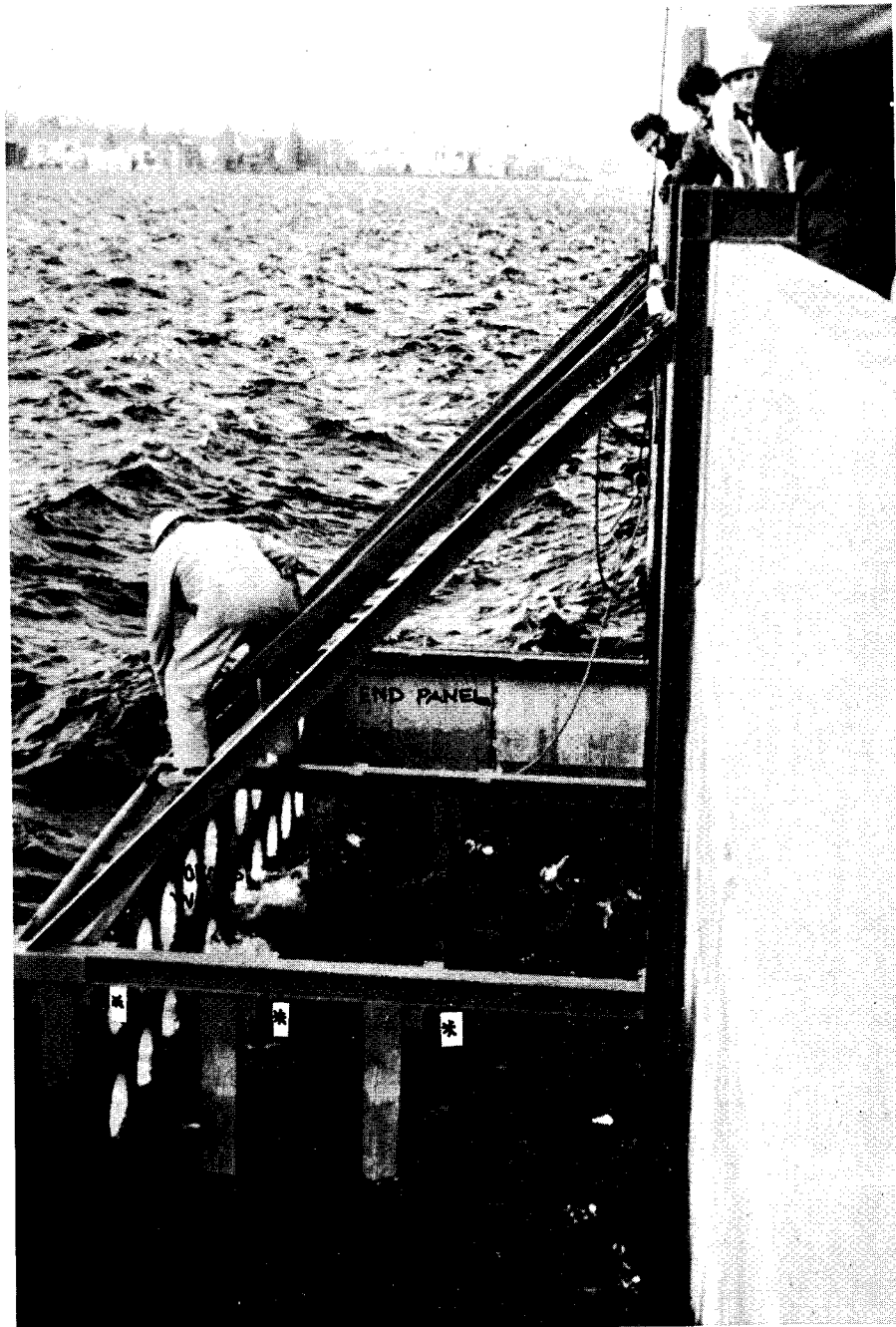
* TEST SECTION CANTILEVER BEAM ASSEMBLY RECEPTACLES
