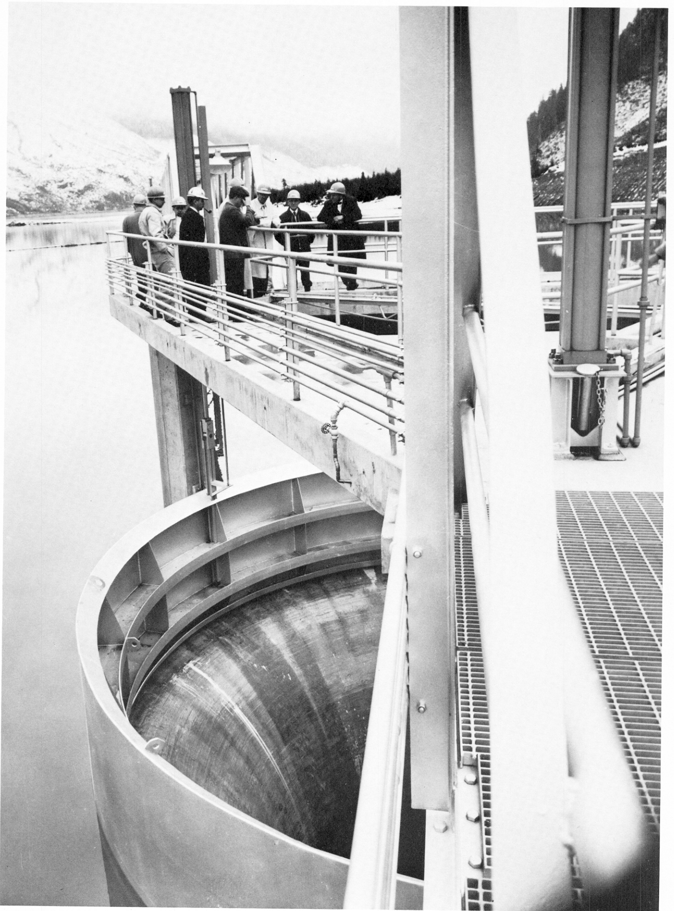
TOLT RIVER DAM SPILLWAY
