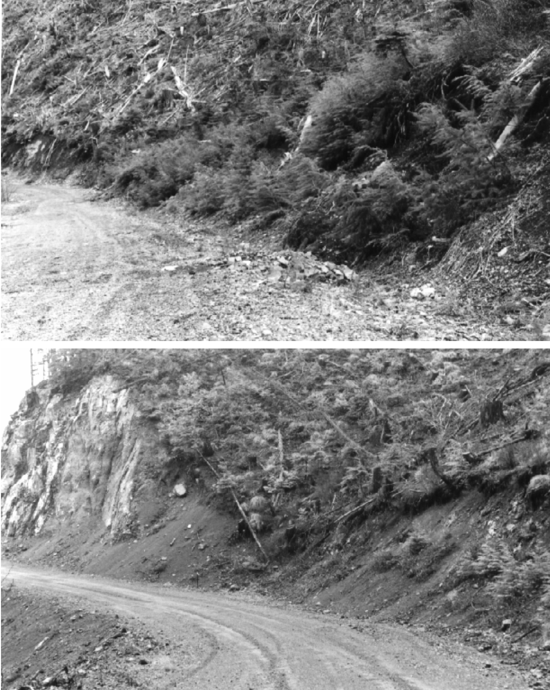
FIGURE 3-12: TWO EXAMPLES OF EXPOSED CUT SLOPES
