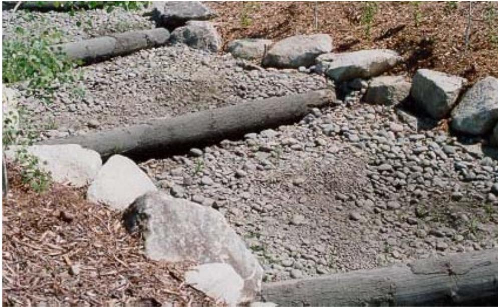
**Figure 6-2:** Typical bed cross-section for the constructed Viewlands swale
