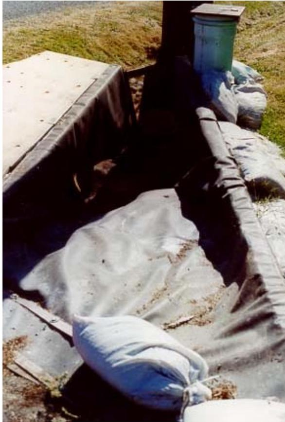
**Figure 4-8:** The constructed stilling basin and stand pipe housing the shaft encoder at the SEA Streets site
