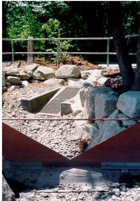
**Figure 3-5:** View of Cell 16 that includes a 120° V-notch weir and the concrete culvert with metal grating (facing downstream towards Pipers Creek)
