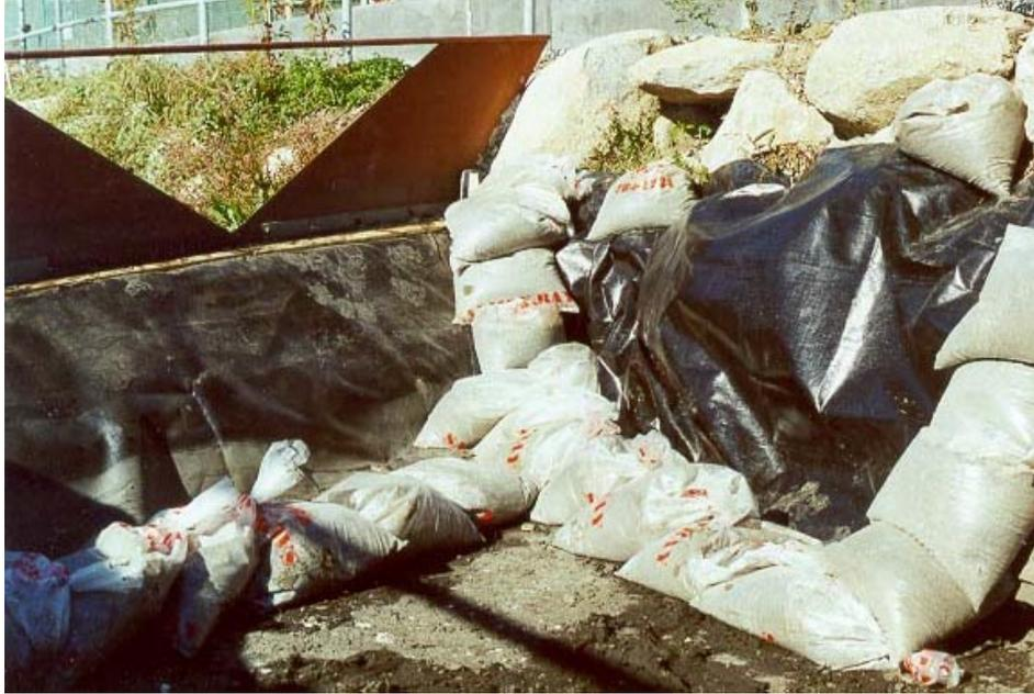
**Figure 7-4:** Remedial measures taken in October 2000 at the upstream V-notch weir
