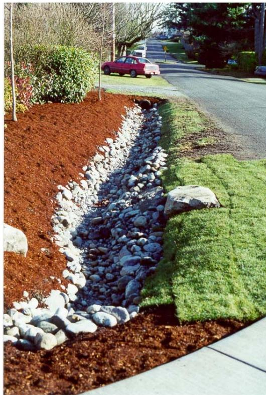
**Figure 7-12:** Swale system that replaced a concrete-lined open drainage ditch
