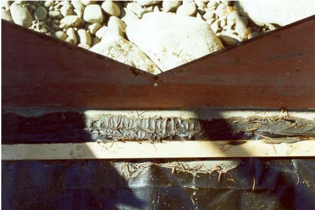
**Figure 7-1:** Environmental deterioration and geometric constraints of the V-notch weir
