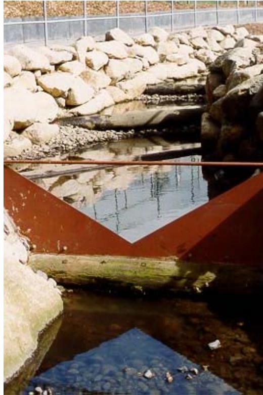
**Figure 4-7:** The downstream V-notch weir with Cells 15 and 16 filled (facing upstream towards NW 105<sup>th</sup> Street)
