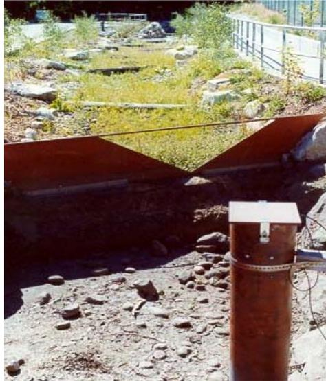
**Figure 3-4:** View of Cell 1 that includes the stand pipe housing the flow monitoring equipment and a 120° V-notch weir (facing downstream towards Pipers Creek)
