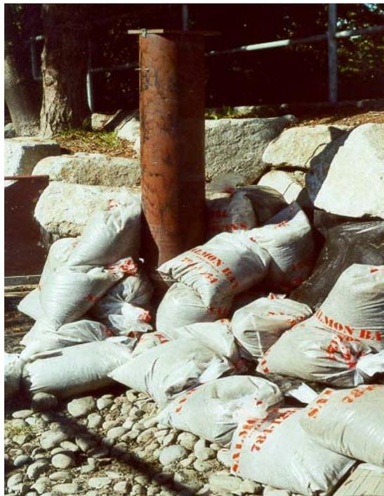
**Figure 7-5:** Remedial measures taken in October 2000 at the downstream V-notch weir
