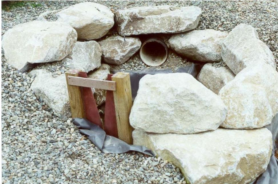
**Figure 4-9:** Construction of the new monitoring stilling basin at the SEA Streets site
