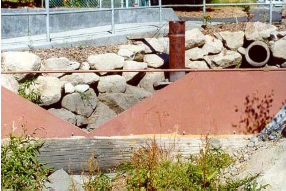
**Figure 4-6:** The upstream V-notch weir, standpipe, and influent pipe (facing upstream towards NW 105<sup>th</sup> Street)
