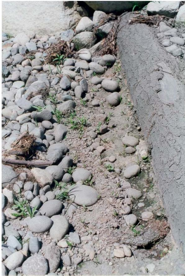
**Figure 6-1:** Scouring downstream of each log weir from 6 to 8 in (15.2 to 20.3 cm)
